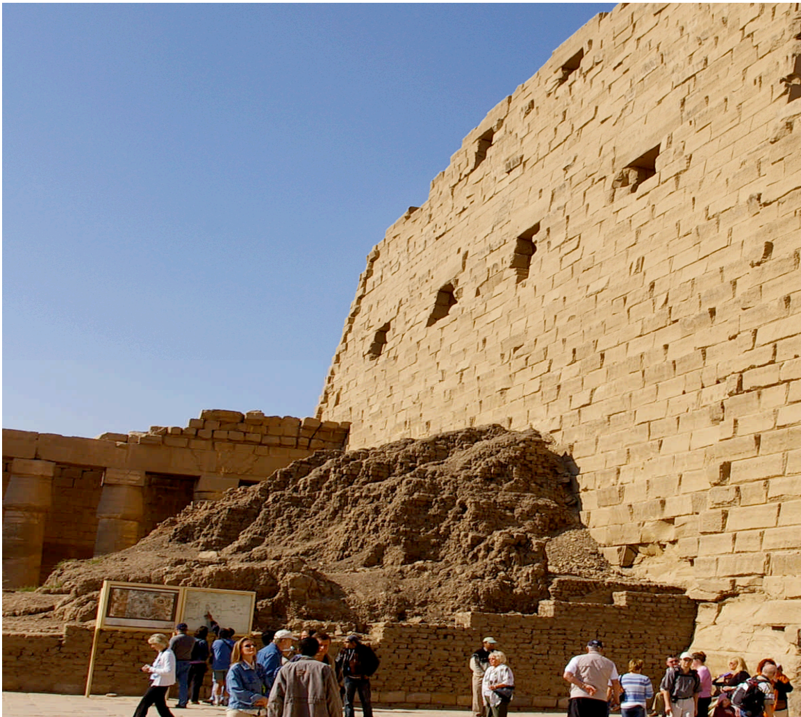
Fig. 4. Remains of construction ramp at Karnak Temple.
